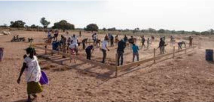
**Worksite Shift:** The work consists of digging the foundation, sifting sand, mixing concrete, making bricks, carrying water, and tying rebar. It is physically hard work. Everything is done by hand, and you will probably have blisters and sore muscles.
